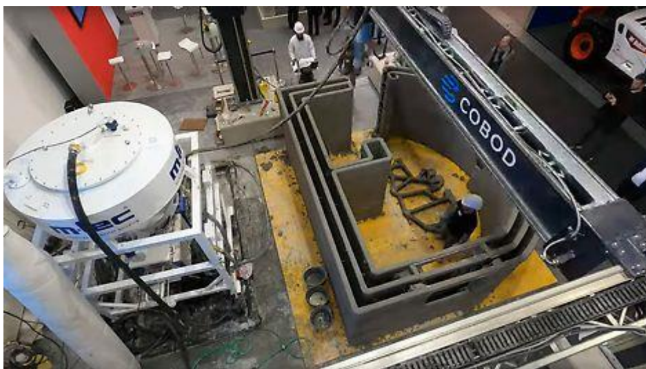
Figure 14 3D printed wall printed with BOD2 printer
