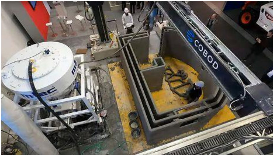
Figure 12 3D printed wall printed with BOD2 printer
